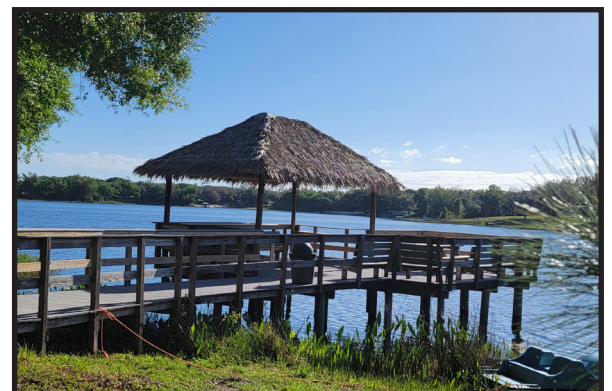
The Farquhar Overlook deck received a covered area and adjustable railing for accessible fishing.
