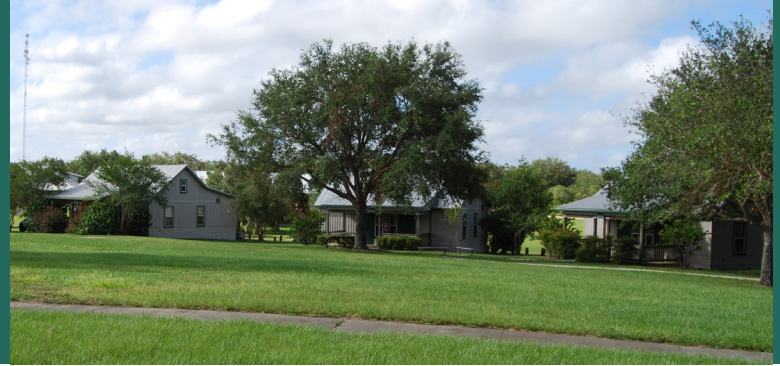
Three of the seven Hillside cabins. Four units still to be built.
